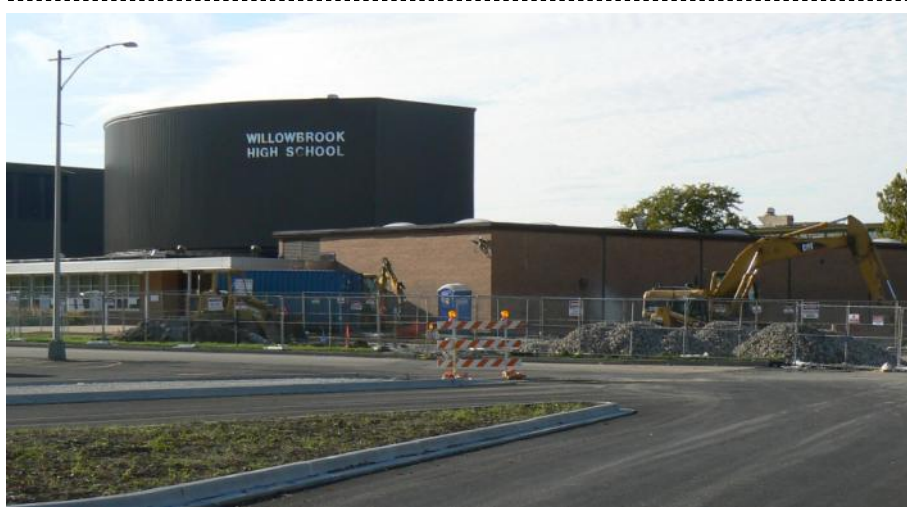
Financial support from Local 571’s COPE fund and the DuPage District 88 Teachers Council helped the district’s “Building The Future” campaign mount a successful referendum. Voters approved $110 million in bonds that are now paying for major renovations and new additions to Addison Trail and Willowbrook High Schools. October foundation work expanding Willowbrook’s music wing is pictured.
